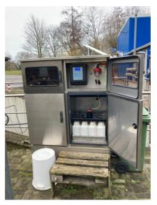
Figure 9 -Automated Sampling Device at the WWTP Aachen Soers (courtesy of F. Joerens, Wasserverband Eifel-Rur)
