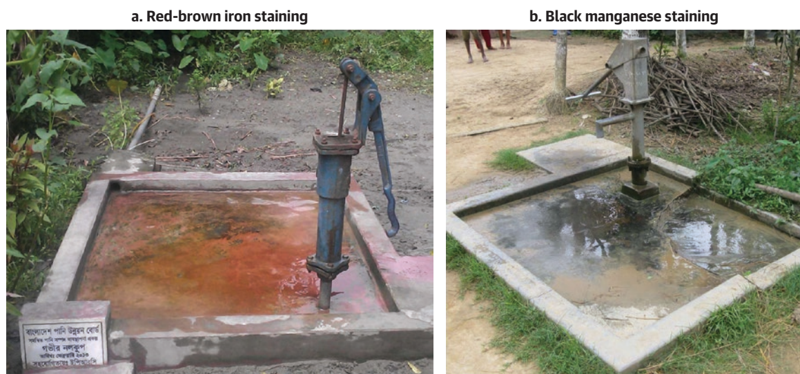
PHOTO 4.1. Examples of Iron and Manganese Staining at Handpumps
